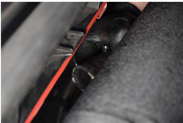
45. Install the recirc pipe onto the intake pipe.
